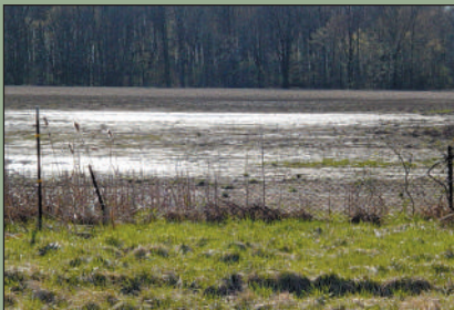
Low permeability and high water table results in ponding.
