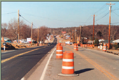
Widen and extend roads and upgrade intersections
